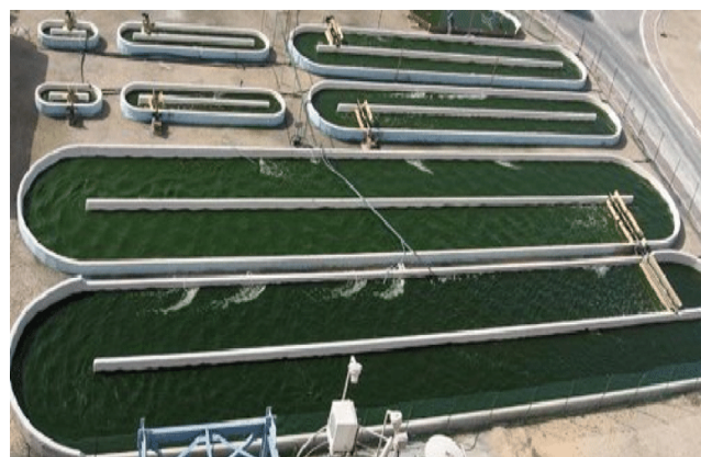
Figure 1.2 Open raceway microalgae production pond adapted from (Kumar and Jain, 2014).
