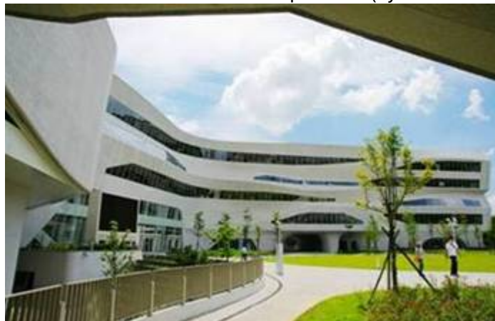
Photo 1: Outward look of NLPI new pavilions (by this research)
