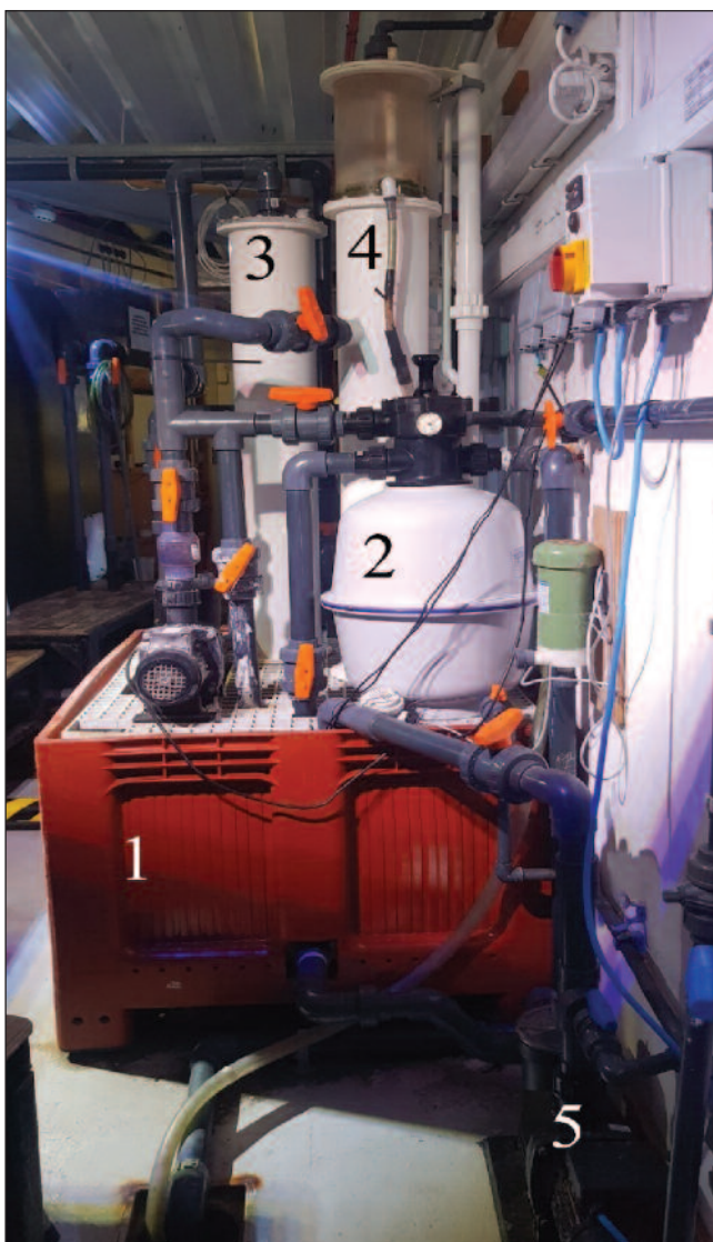
Figure 3. A view of the LSS for the Chrysaora spp. kreisel systems. Within this image you can see; 1 – sump; 2 – sand filter; 3 – biological trickle tower; 4 – protein skimmer, a rapidly aerated body of water in which foam fractionation occurs, removing proteinaceous waste from the water; 5 – circulation pump that feeds the chiller loop.
