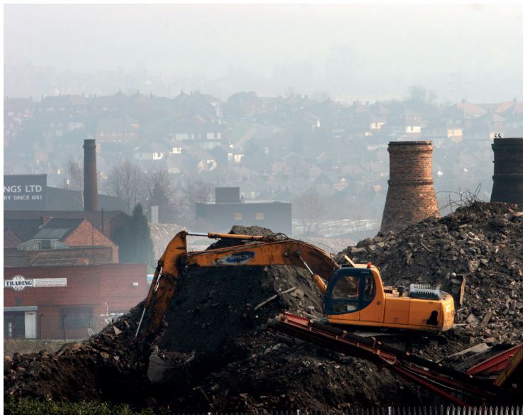
Figure 10: Demolition in Stoke-on-Trent (image ©Ploppy/Alamy Stock Photo)
