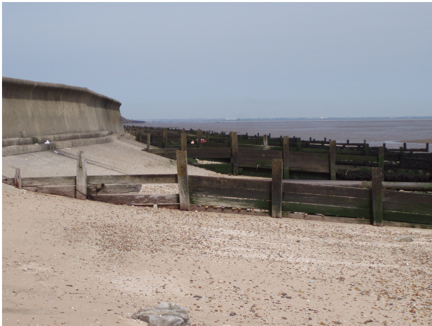
Fig. 13. Holding the line - Coastal zone narrowing is probable where the policy is to 'hold the line' (e.g. Minster, Leysdown to Shellness.)
