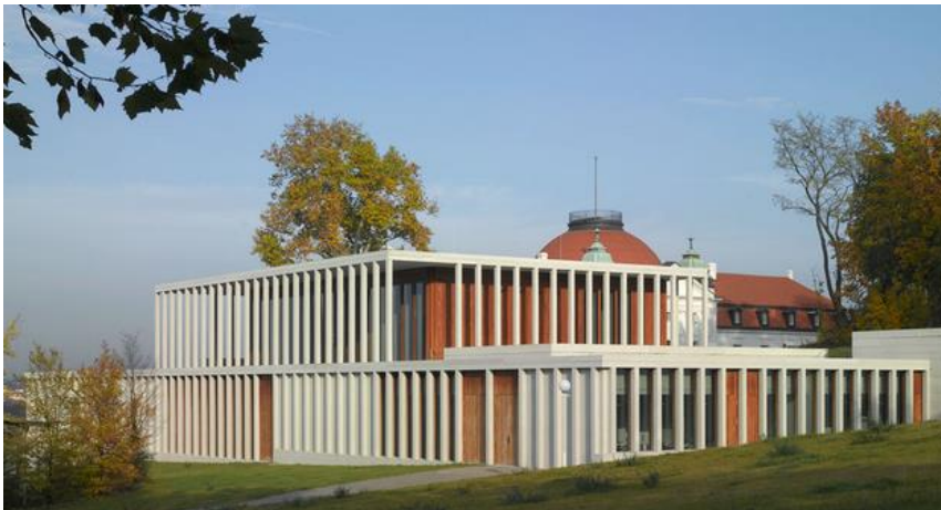
photograph 1 Museum of Modern Literature, Marbach Am Neckar, David Chipperfield, Architects, 2007 RIBA Sterling Prize Winner
