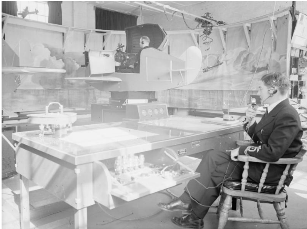
Figure 4. Edwin Link's Blue Box Flight trainer (credit: British Fleet Air Arm Station, 1943). 9
