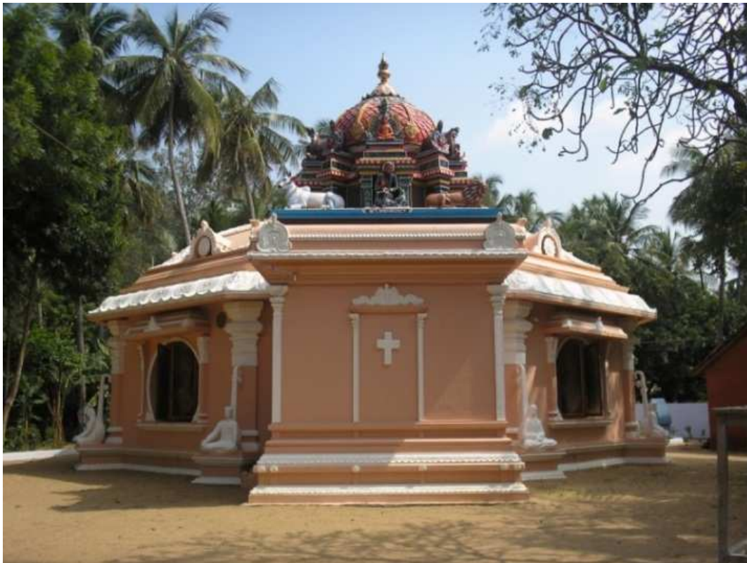
Figure 5 The square part of the building, with the Cross on it, incorporates Abhishiktananda's chapel. Image: author's own (2010)
