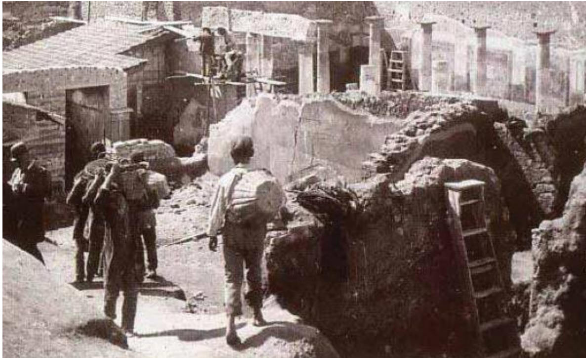
Figure 20. Excavation in Via dell'Abbondanza directed by Spinazzola, Nappo (1998)
