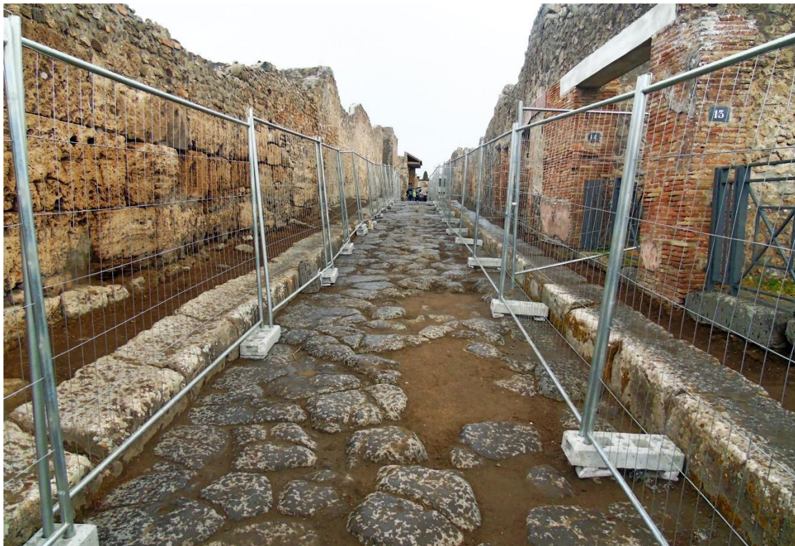
Figure 47. Conservation work and the resulting barriers in Pompeii. This can have a negative impact on the visitor’s perceptions of the site if not properly explained, student own image (2010)
