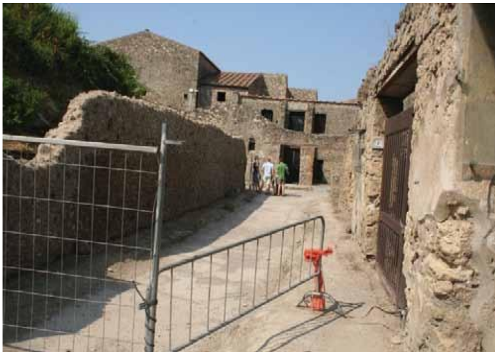
Figure 39. Visitors by the House of the Meander. The barricades in the foreground had been moved by the visitors to get access to the house, which was closed for restoration, Student own image (2017)
