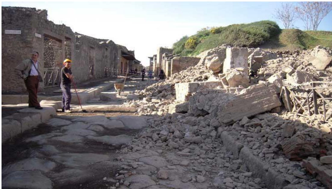
Figure 37. A collapse in Pompeii at the end of the 1990s (Via dell'Abbondanza), Wallace-Hadrill (2012)
